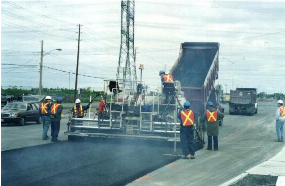
PHOTOGRAPH 3: Standard Asphalt Spreader Laying Performance-Graded Asphalt Cement Recycled Hot Mix
